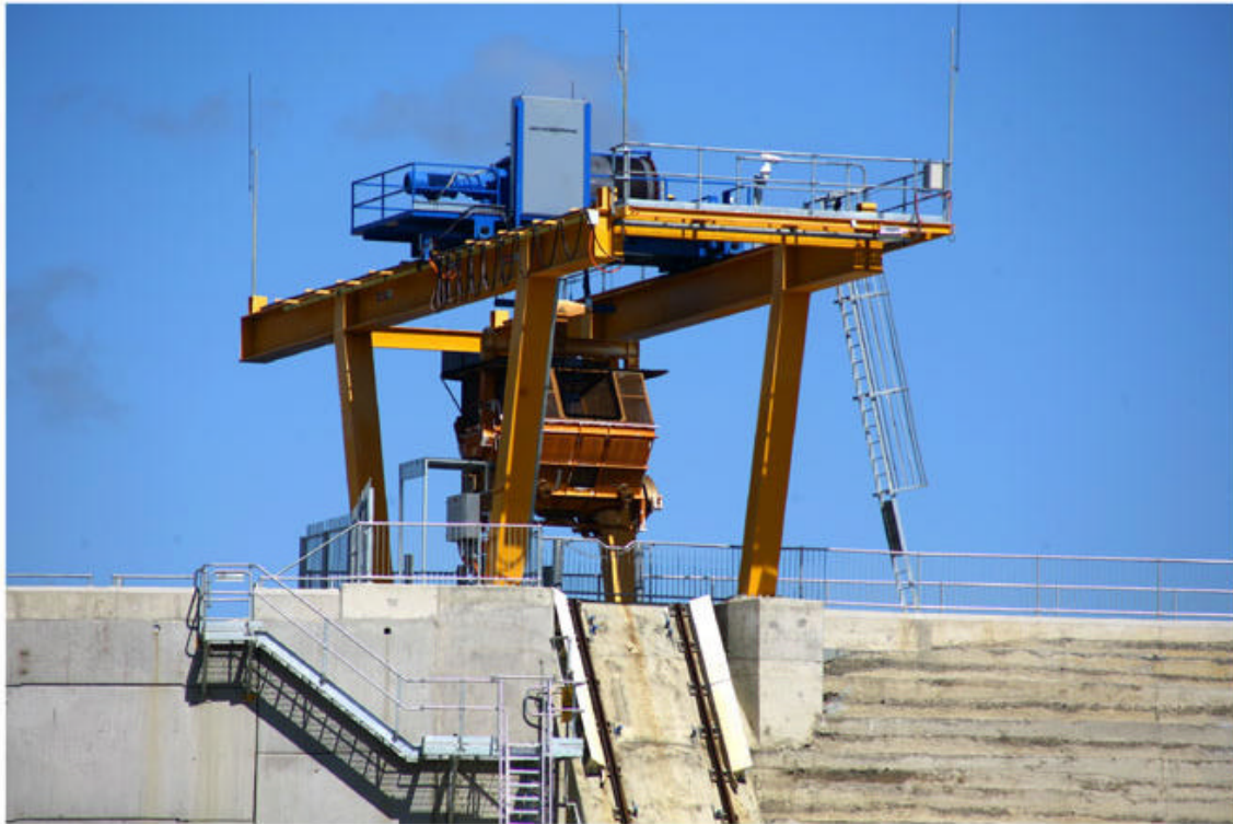
Image 8: Fishlift not in operation on top of Paradise Dam wall. Taken by Arkin Mackay, August 2006.
