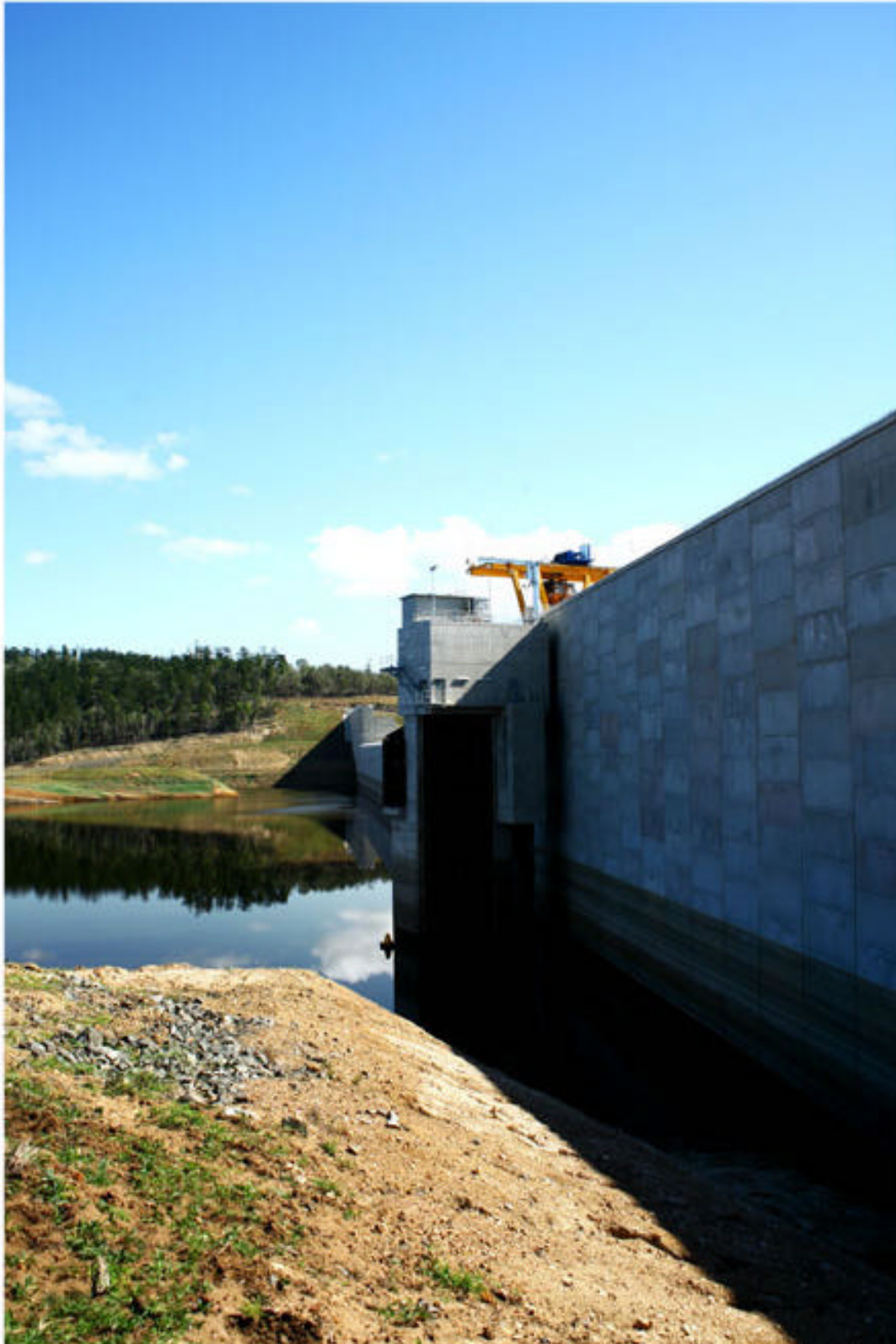
Image 2: Paradise Dam wall showing dam reservoir. Main structure in mid-ground is the main water outlet tower (downstream fishway is barely visible in front of it). Fish hopper visible as yellow structure on top of dam wall. Taken by Arkin Mackay, August 2006.
