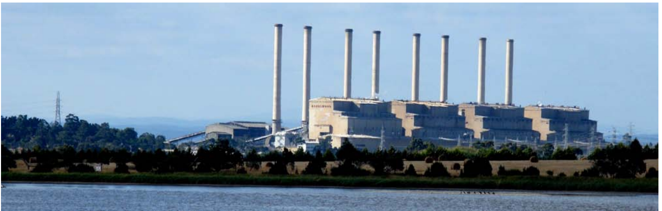
Figure 5: Picture of Hazelwood Power Station, Victoria. Photo by nipper30 from GoogleEarth.
