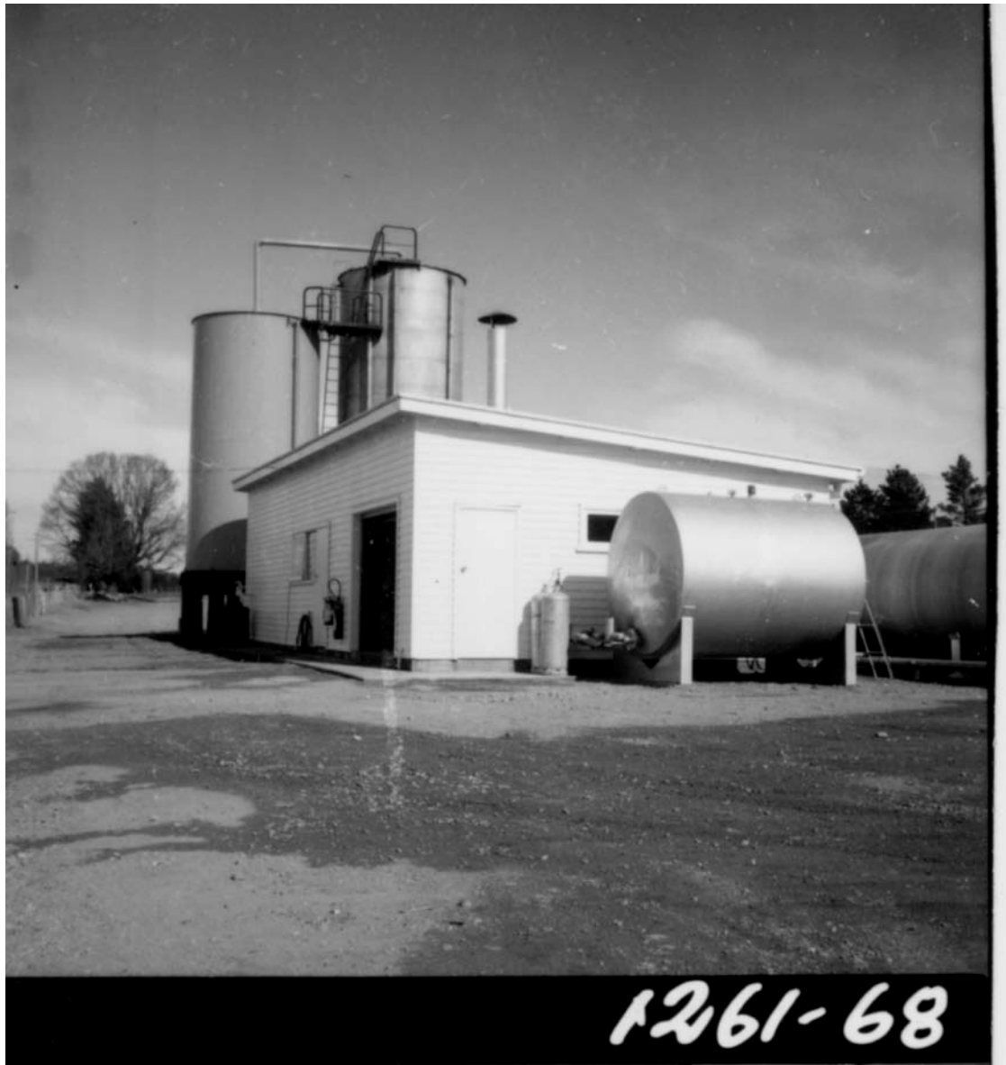
Figure 3: Timber treatment works at Martin Street, Armidale ca 1968. Note that part of the 75 foot cylinder for timber impregnation shown in Figure 5 is visible on the right of this photograph. Source: Armidale City Council file
