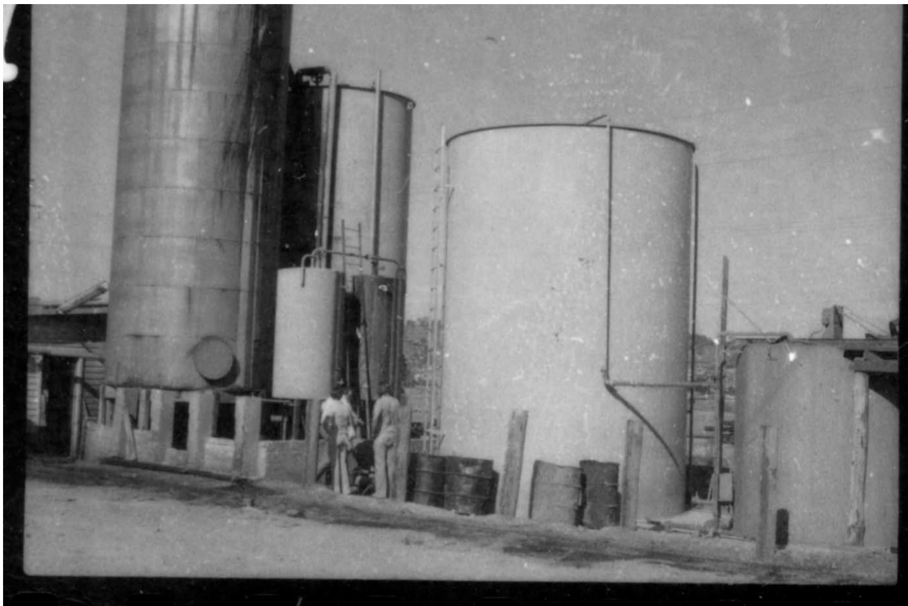
Figure 4: Storage tanks at timber treatment works at Martin Street, Armidale ca 1968
