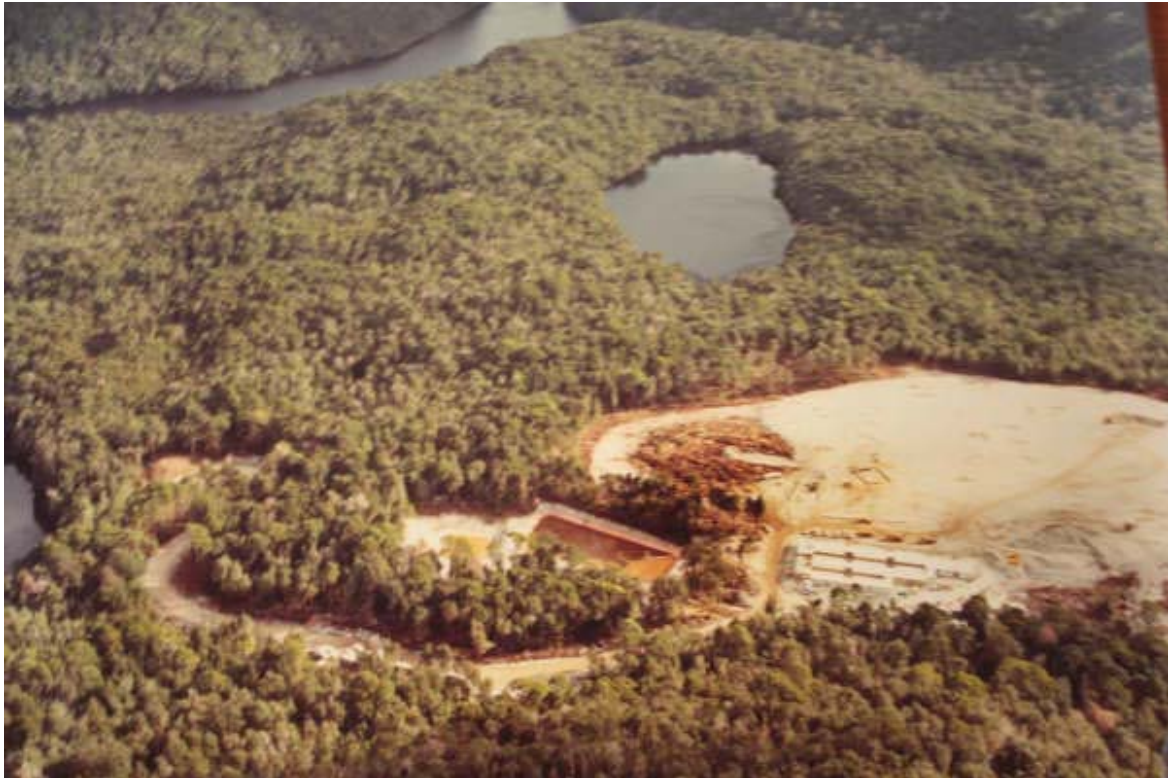
Photograph 1 – Construction site of dam 24 May 1983
