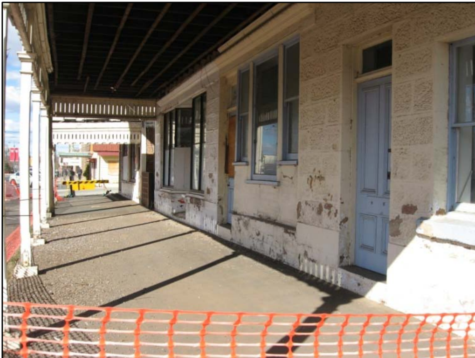
Figure 4: View of ground floor from Fitzroy Street footpath
