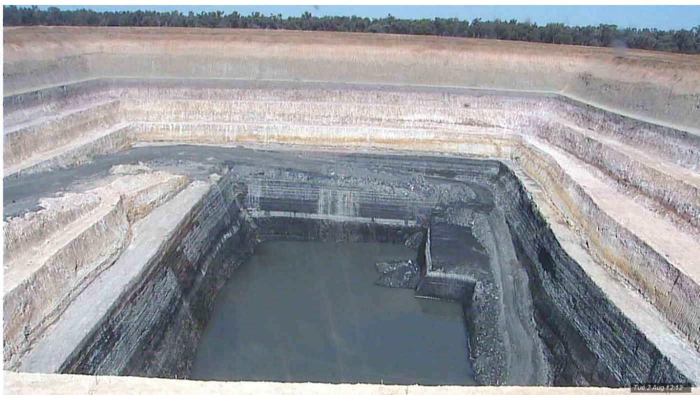
Plate 4: Tuesday 2 August - 2 weeks after perimeter bore pumps switched off
