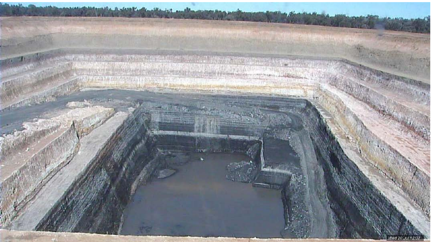
Plate 2: Wednesday 20 July – Perimeter bore pumps switched off
