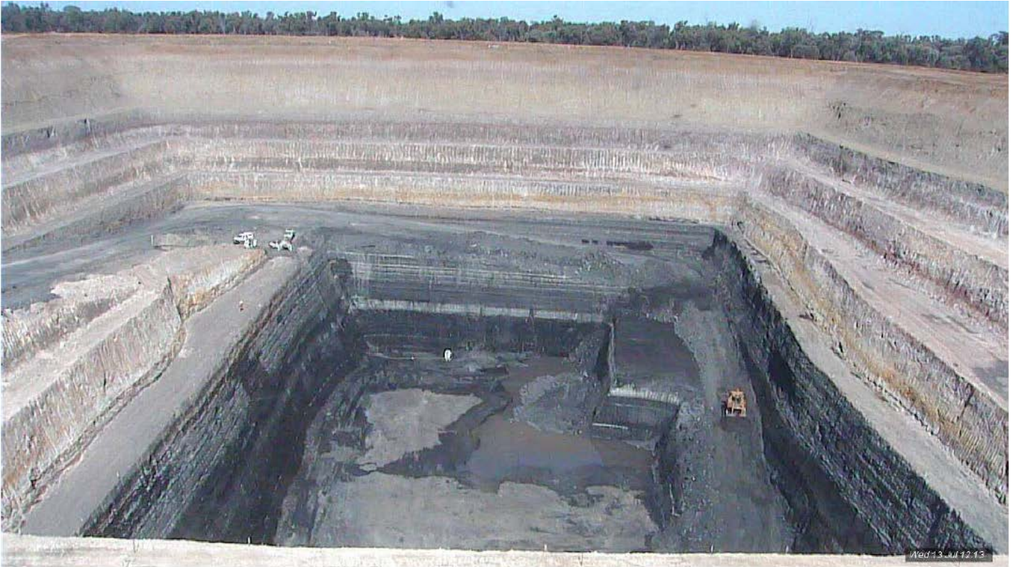
Plate 1: Wednesday 13 July – Sump pump switched off, perimeter bore pumps remain operational
